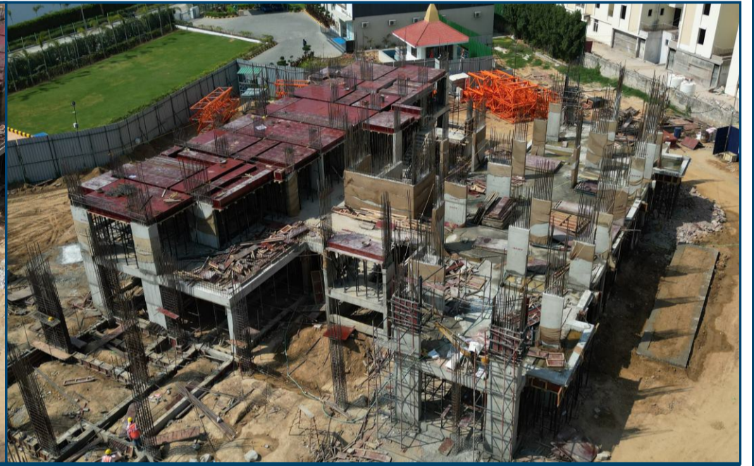
First Floor Roof Casting-Work in Progress
