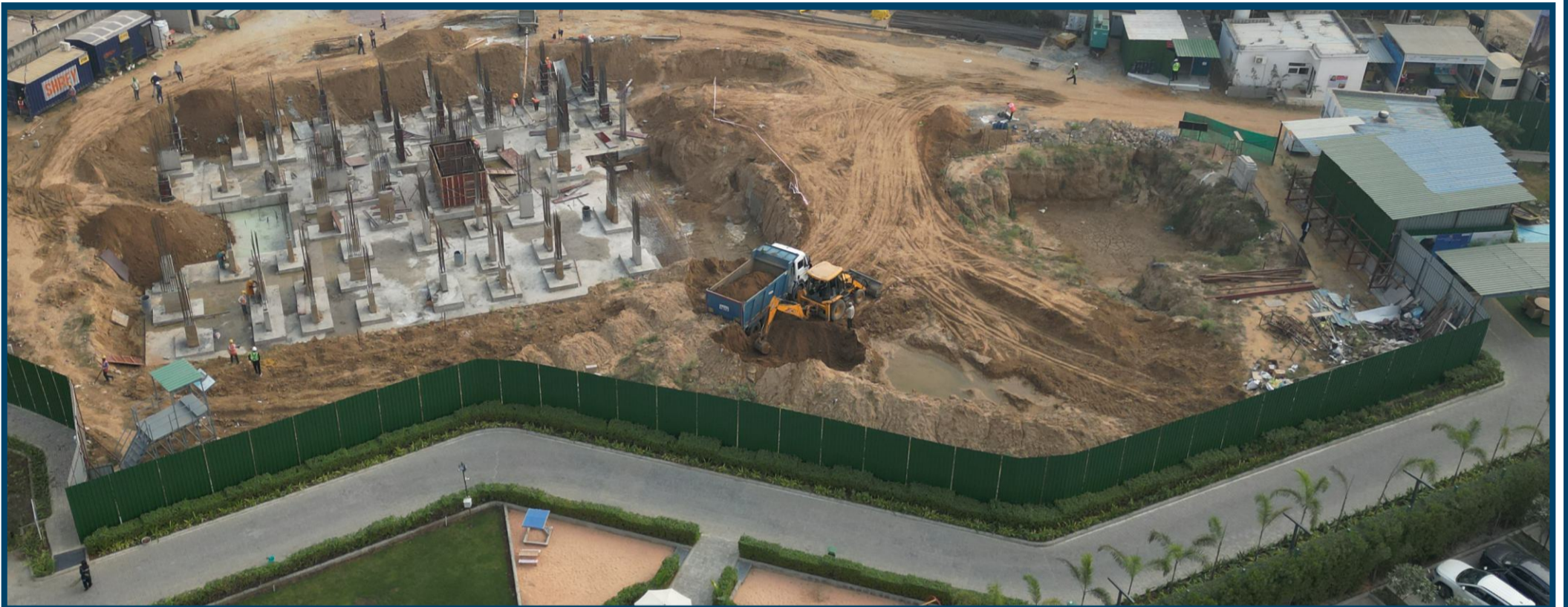
Foundation Work In Progress
