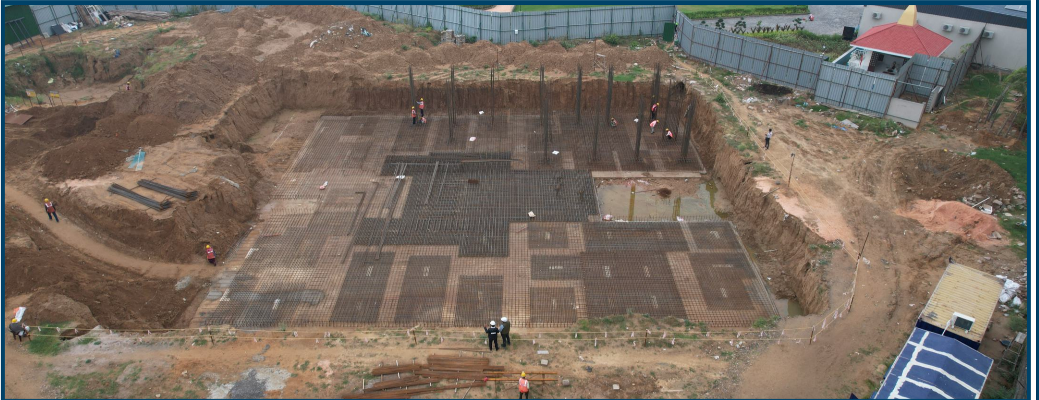
Foundation Work In Progress
