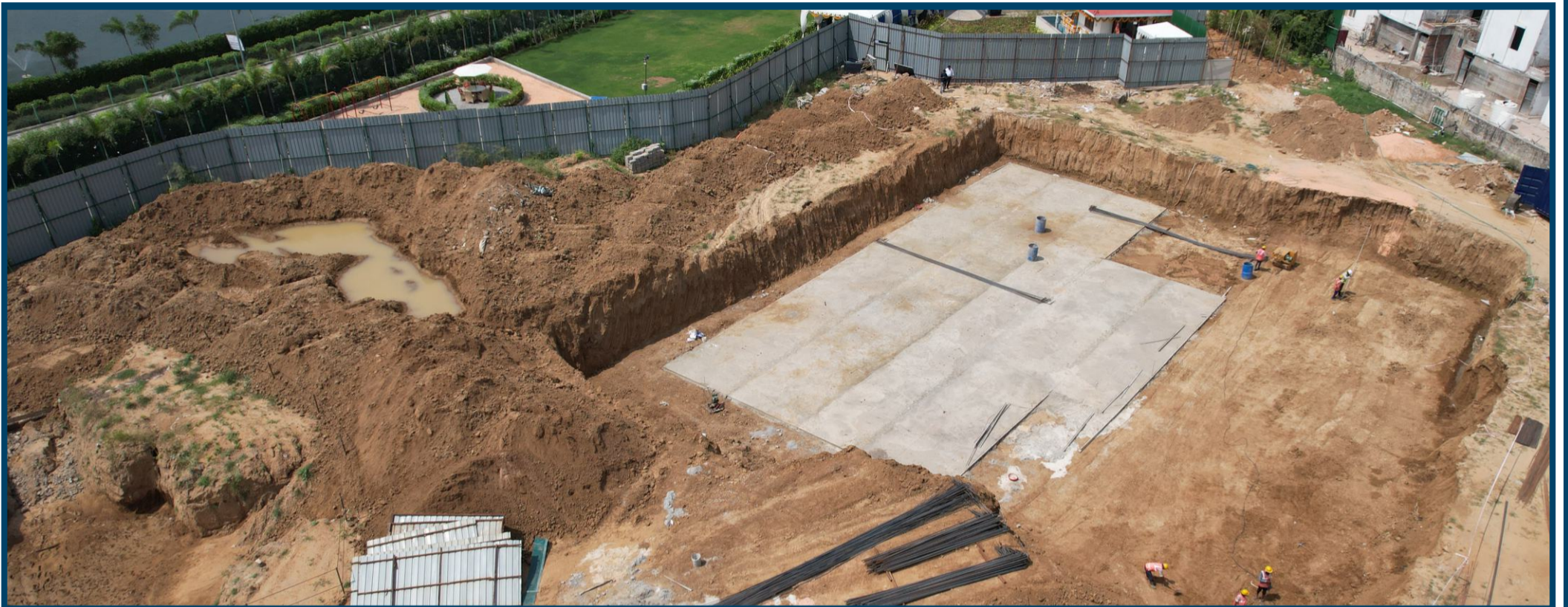
Foundation Work Started
