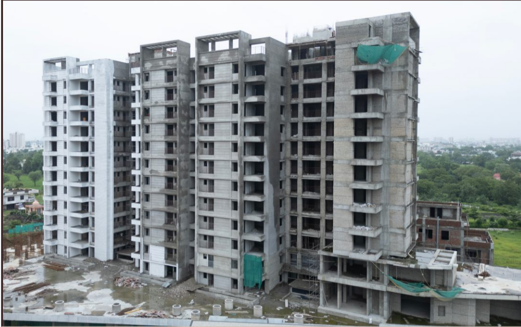
ON GOING- PAINT WORK
