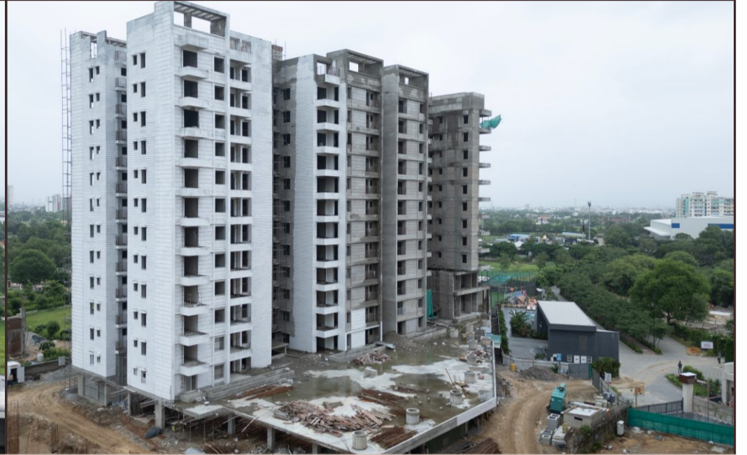
ON GOING- PAINT WORK
