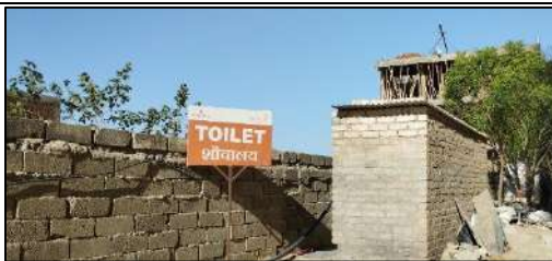
Toilet facility for workers
